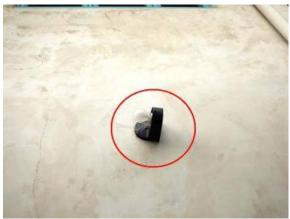
A missing receptacle cover plate was noted at the garage southwest interior. Some lights were not functional. Recommend replacing bulbs and retesting lights.
