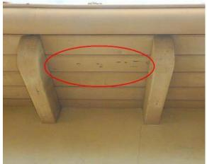
An excessively weathered fascia board was noted between the upper and lower roofs at the upper south portion of the house.
