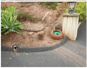
Bare dirt was noted at various places at the slopes. Erosion has occurred in various places.
