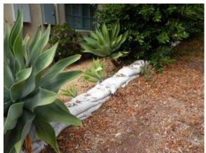
Bare dirt was noted at various places at the slopes. Erosion has occurred in various places. Recommend planting drought tolerant foliage to help prevent erosion.
