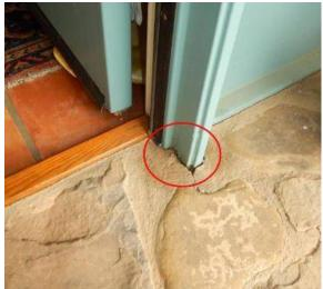
High thresholds were noted at the living room and family room. High thresholds can be trip hazards and are not to current standards.
