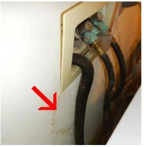
Excessive mineral deposits and evidence of leakage were noted at the laundry supply valve. Recommend improvements be made by a licensed plumbing. A new laundry supply valve and hoses have been installed.
