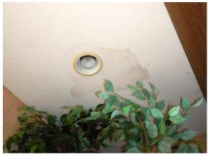
Moisture stains and damage were noted at the upper hallway ceiling and wall toward the rear of the building.
