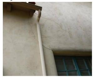
Open cracks were noted in various places at the exterior walls. Recommend sealing open cracks to help prevent water intrusion.
