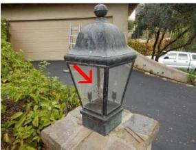
A displaced light fixture with a missing globe was noted at the north exterior.
