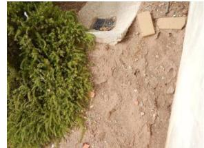
Bare dirt was noted at various places at the slopes. Erosion has occurred in various places.
