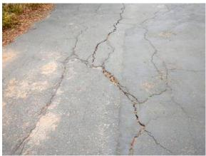
Open cracks were noted at the common driveway.
